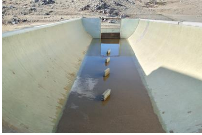
Fig.3 View of the installed plates
